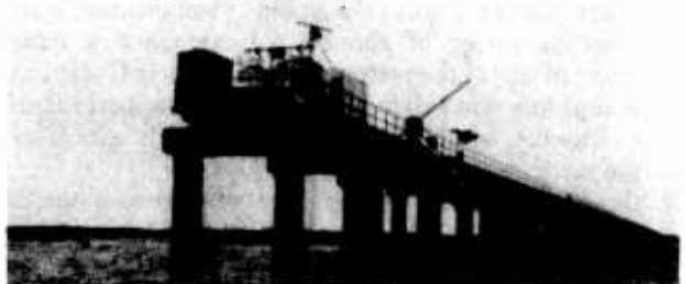
Fig. 1. CERC field research facility pier.
