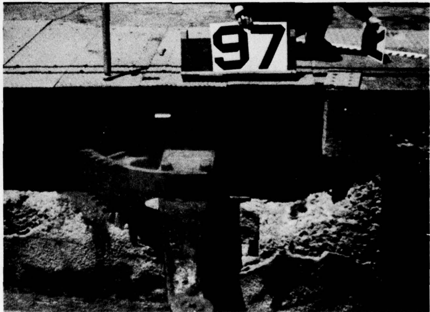
b. Lock and Dam 3, Monongahela River, Pennsylvania
