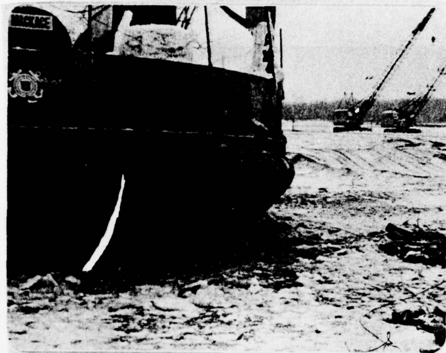
MACKACE ON HOVER SHOWING RIP IN SEGMENT
