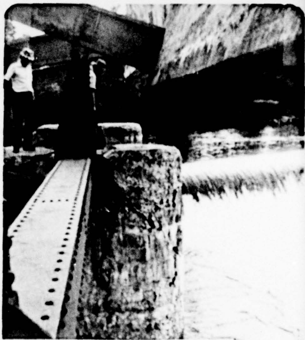
5. Views of second pier from west side showing sheared concrete pier section on both sides. Apparently, crack goes clear through section. Notice double tension rods in right picture located at foot of dam inspector.
