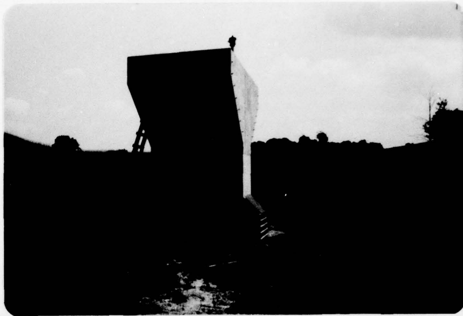
Dam 1 - Principal Spillway Riser Photo #7
