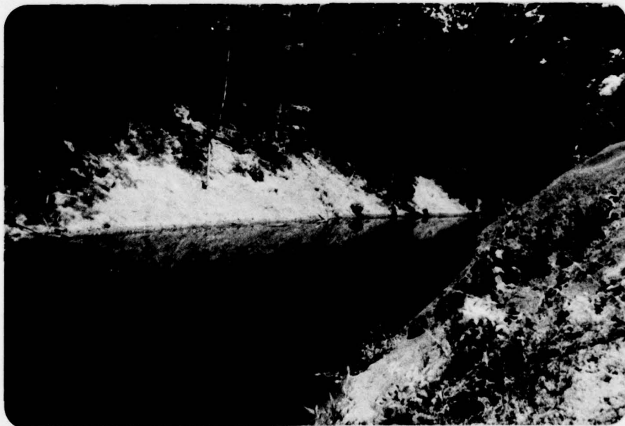
Steep Slopes in Reservoir Area Note Shale Outcrop at Right Photo #14
