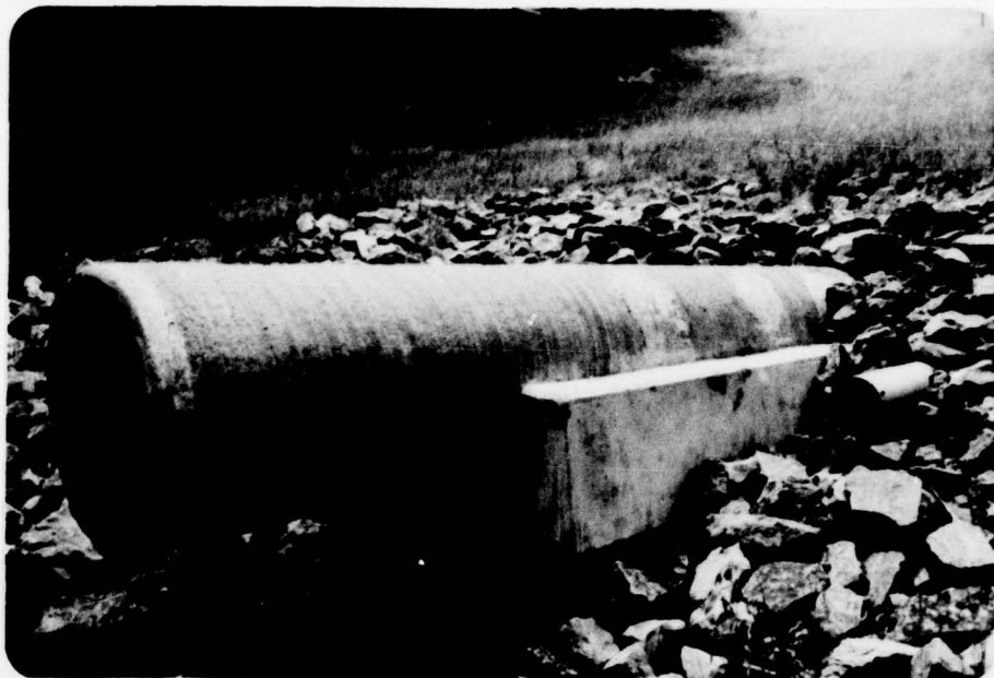
Dam 1 - Principal Spillway Conduit Note Drainpipe Photo #9
