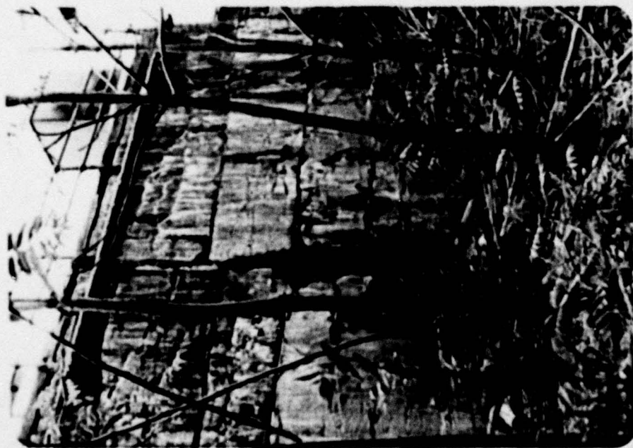
9. Riverside wall of lock shows seepage and advanced concrete surface deterioration.
