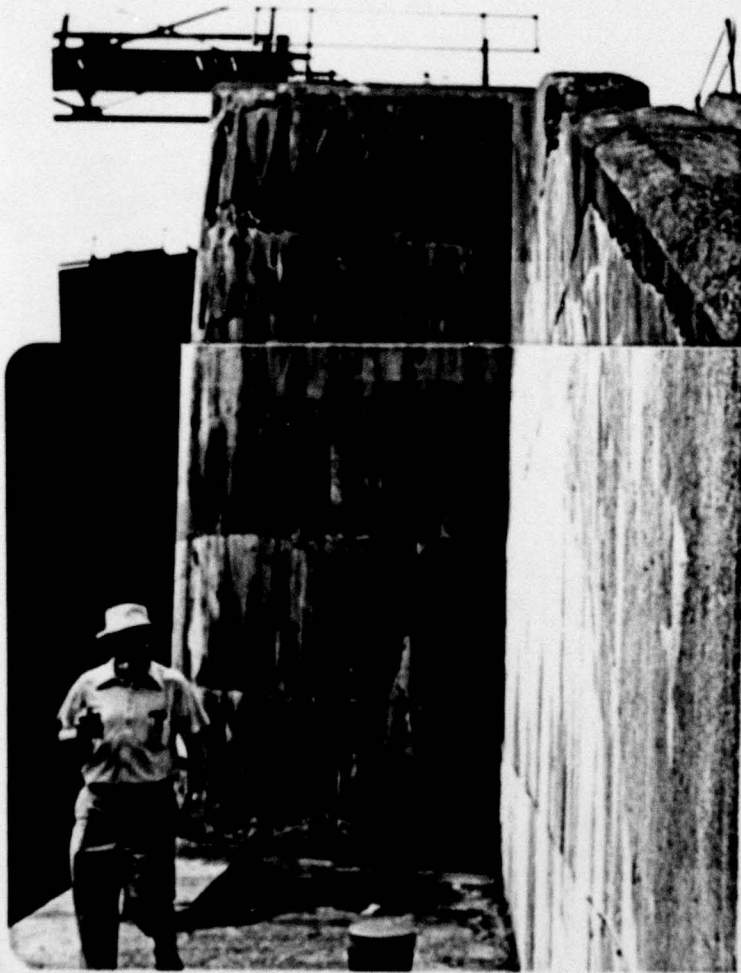
11. Deterioration of downstream walls of lock.
