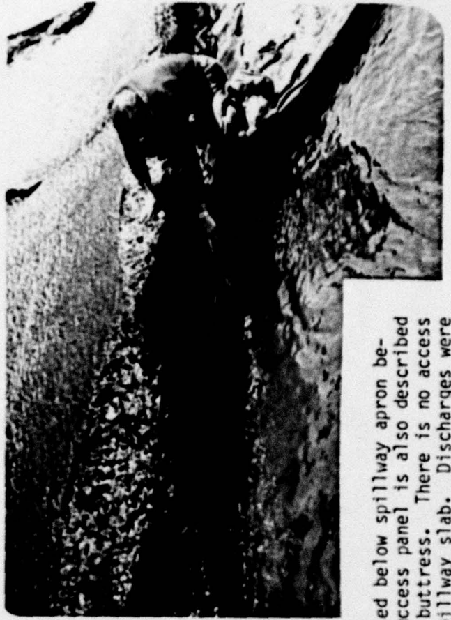
7. Spillway abutment wall on east side of river. Concrete is severely eroded.
