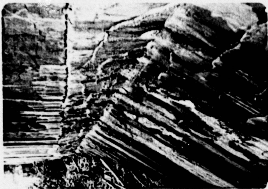
9. Riverside wall of lock shows seepage and advanced concrete surface deterioration.
