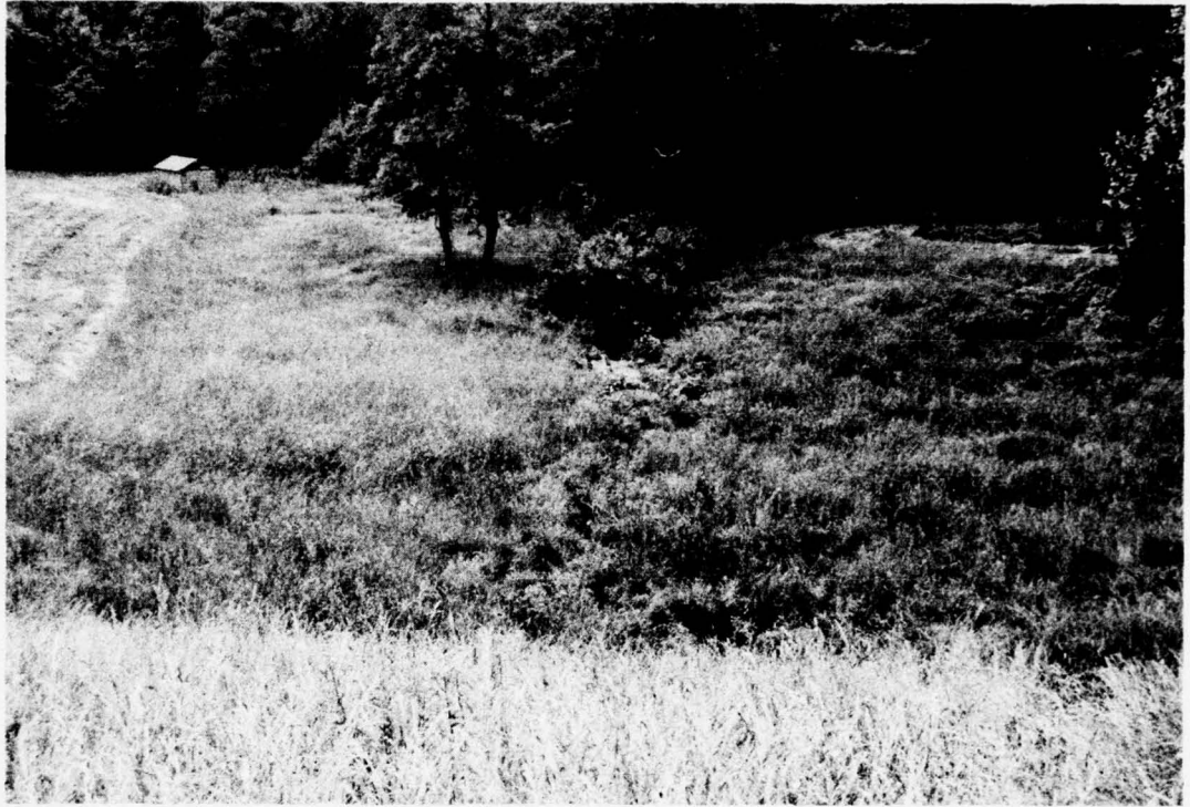
PHOTO 3. View of Downstream Channel from Dam Crest
