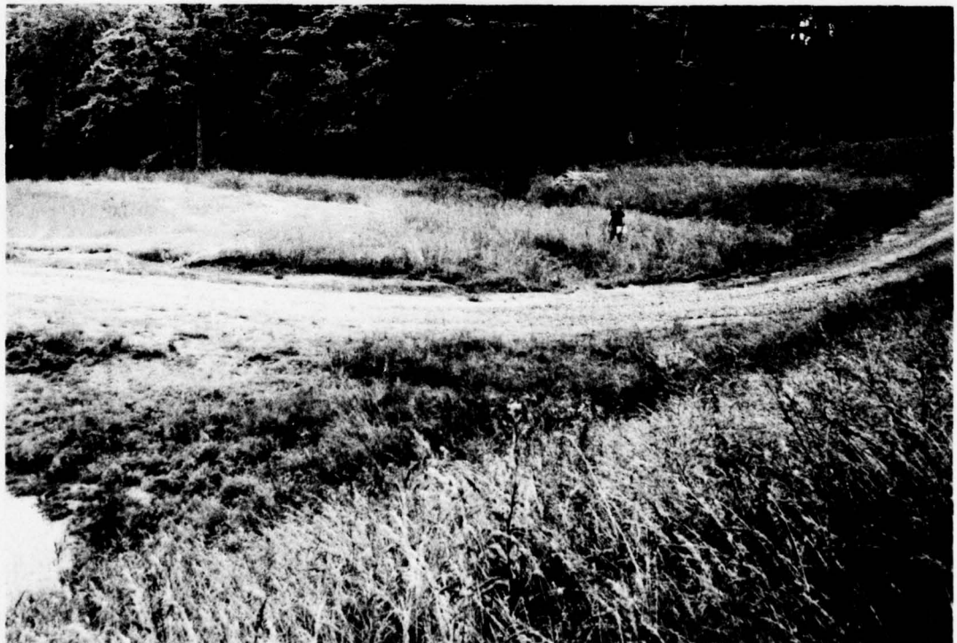
PHOTO 4. Downstream View of Emergency Spillway Channel
