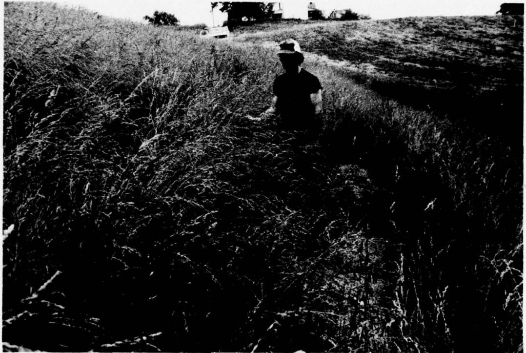
PHOTO 5. Eroded Slump Scarps on the Downstream Embankment
