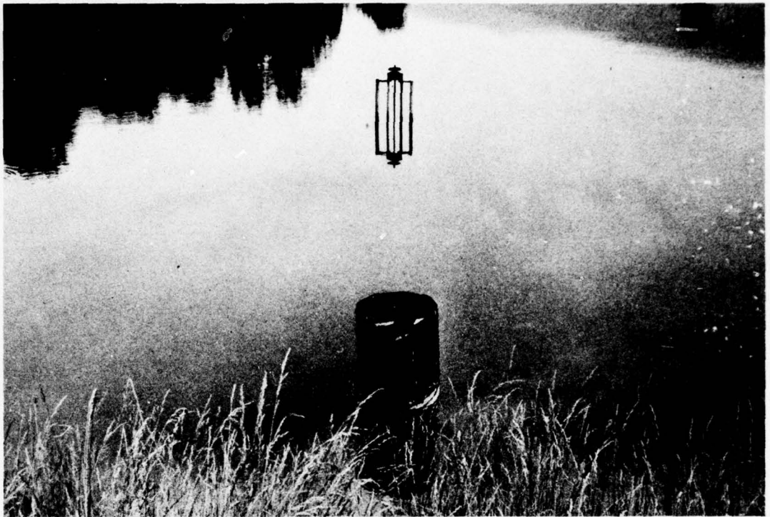
PHOTO 1. Principal Spillway Inlet and Drain Hand Crank
