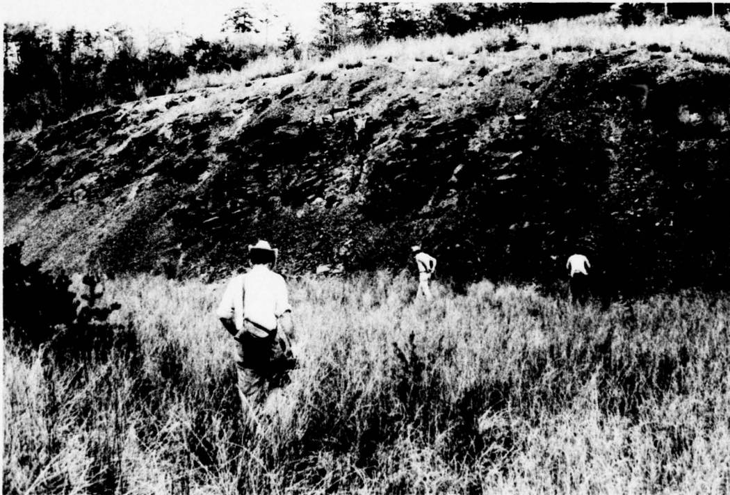
PHOTO 6. Right Cut Slope of Emergency Spillway
