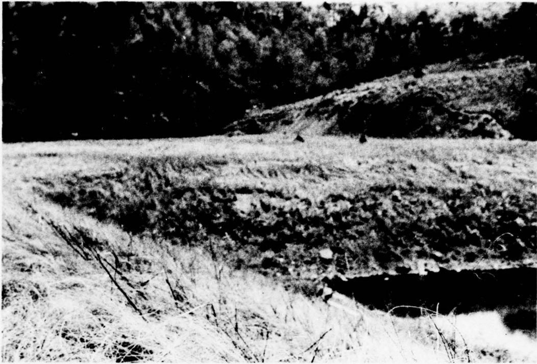
PHOTO 5. Upstream View of Emergency Spillway and Rock Disposal Area
