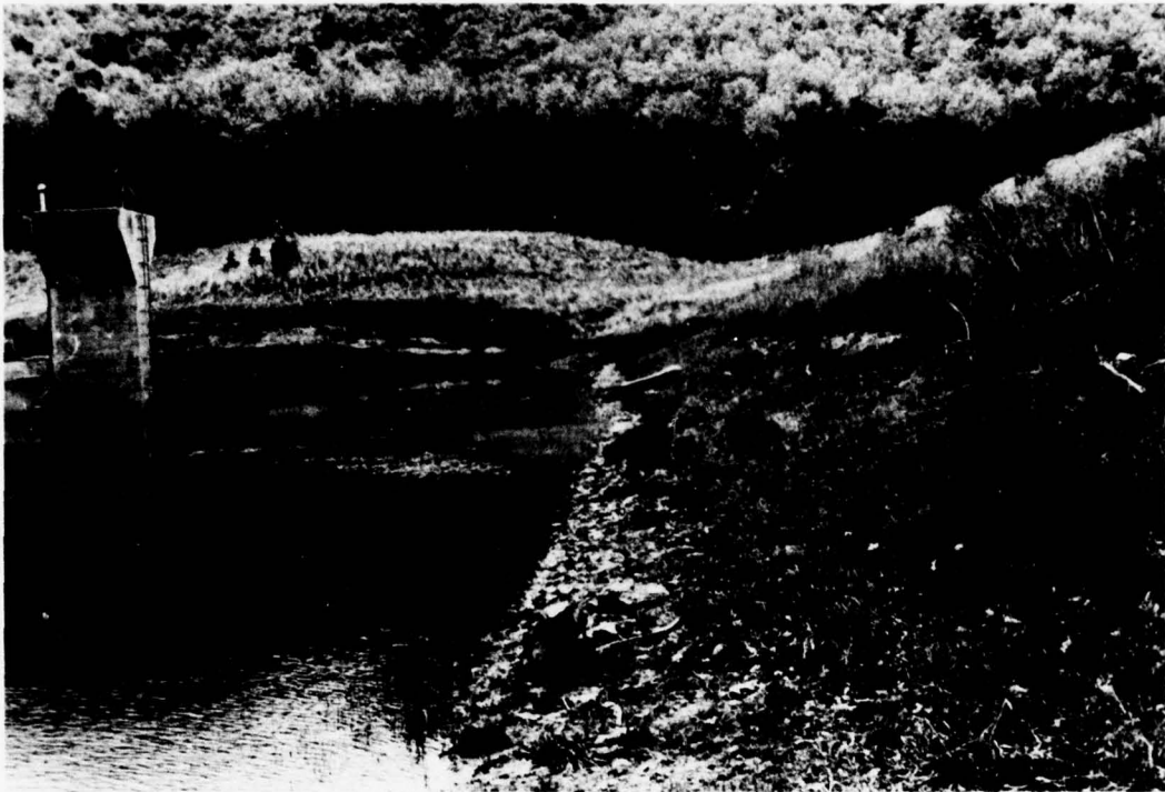
PHOTO 1. Upstream Embankment and Riser
