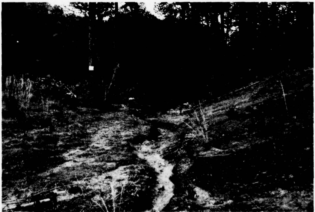
PHOTO 8. Erosion in Discharge Channel of Emergency Spillway
