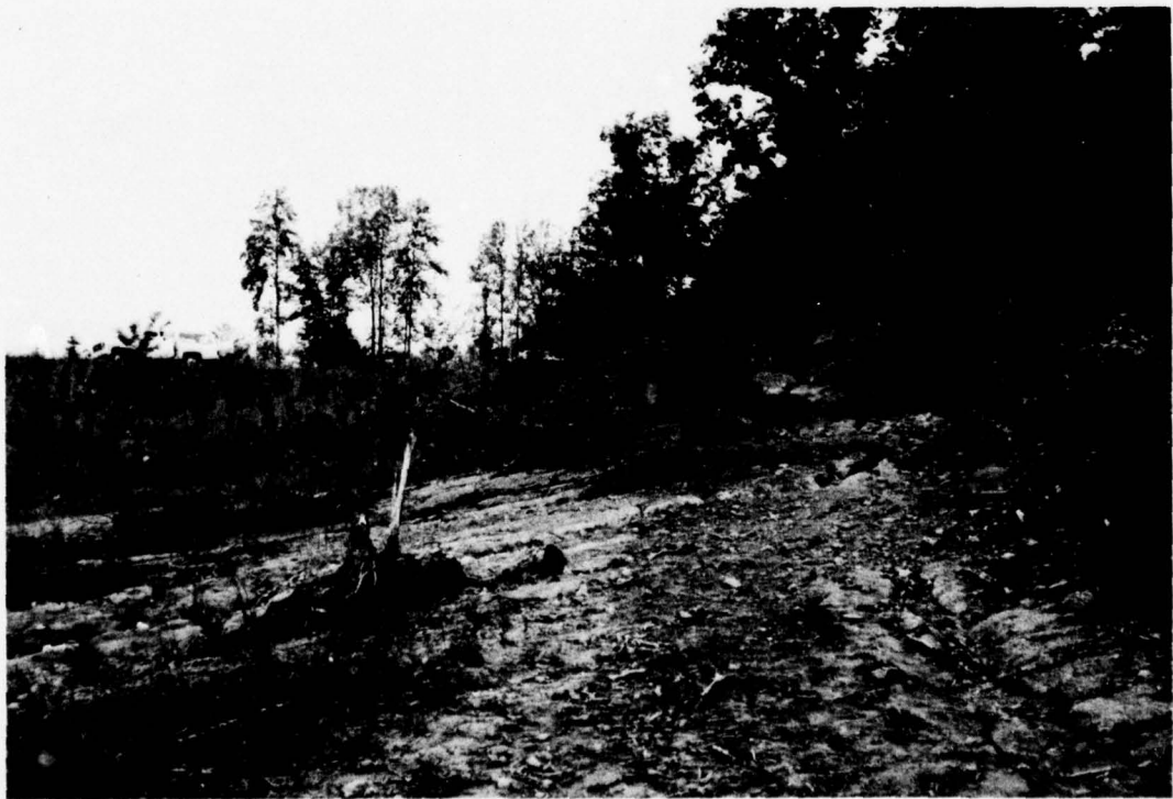
PHOTO 2. Eroded Area on Left Abutment
