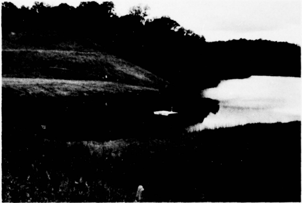
PHOTO 5. View of Riser, Reservoir and Approach Slope of Emergency Spillway (Note Erosion Gullies in Approach Slope)
