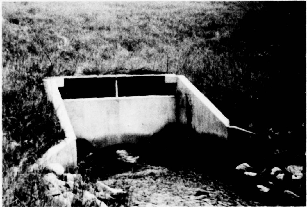
PHOTO 6. Impact Basin with Baffle Wall and End Sill
