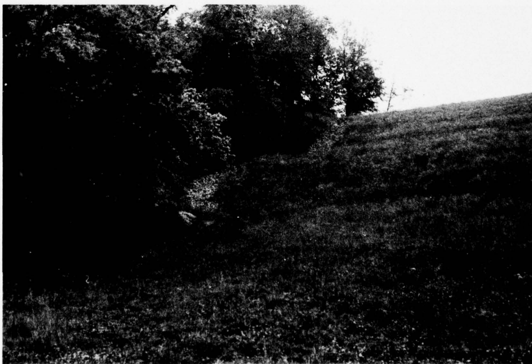
PHOTO 4. Junction of Downstream Embankment and Right Abutment
