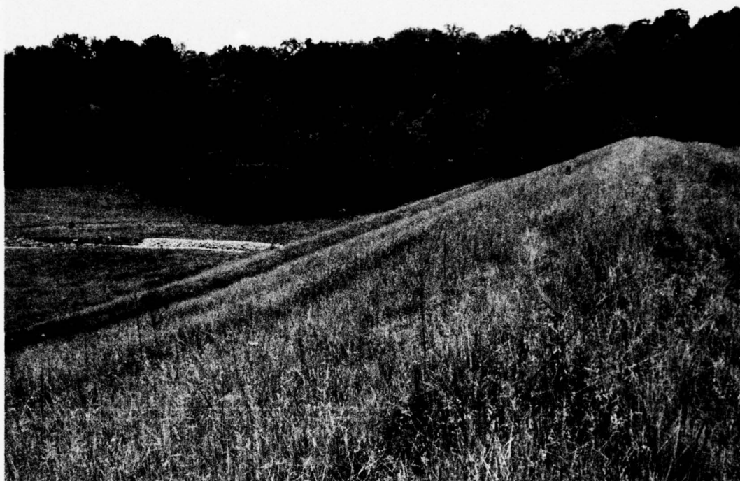
PHOTO 3. Downstream Face of Dam
