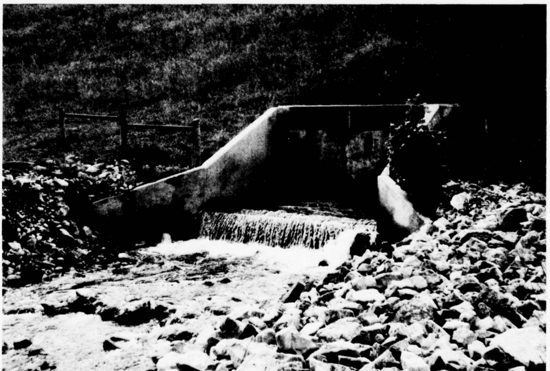
PHOTO 6. Outlet of Principal Spillway, Impact Basin and Riprap-Lined Channel
