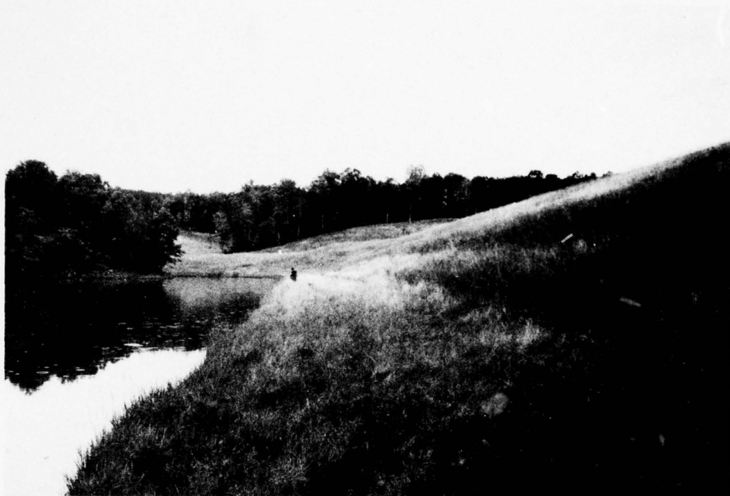
PHOTO 1. Upstream Face of Dam Looking Toward Approach to Emergency Spillway
