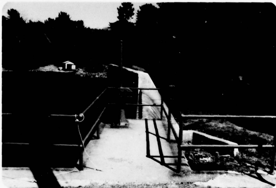
Reservoir Drain Controls, Crest of Spillway and Non-Overflow Section Photo #17
