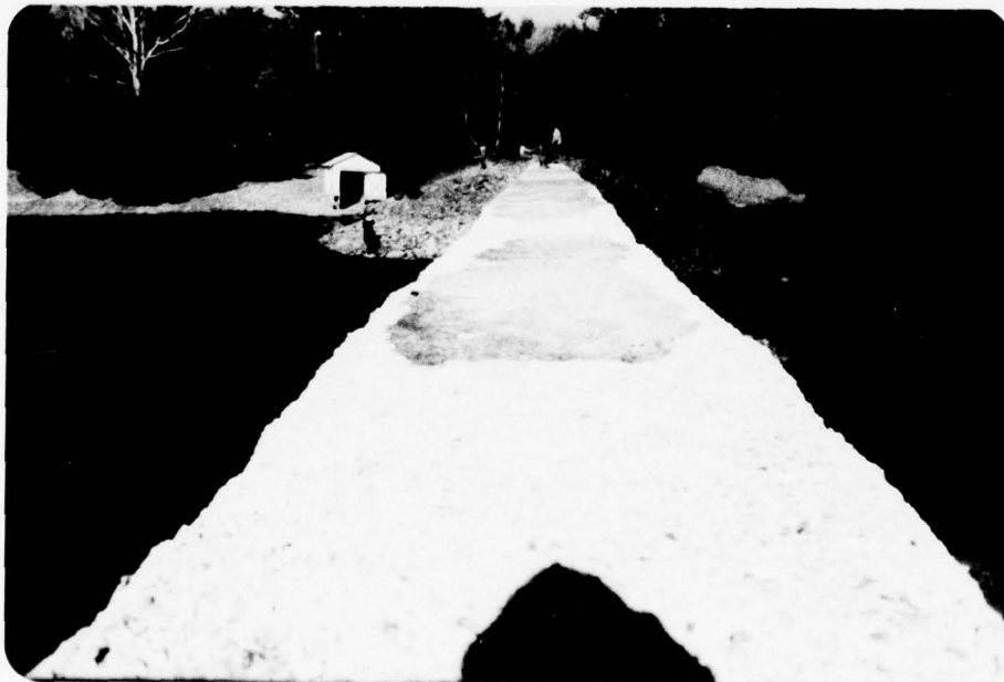
Crest of Non-overflow Section and East Embankment Photo #5
