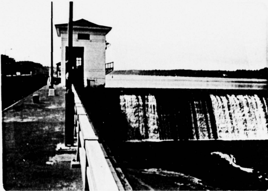
3. Close-up of abutment of dam in south shore.
