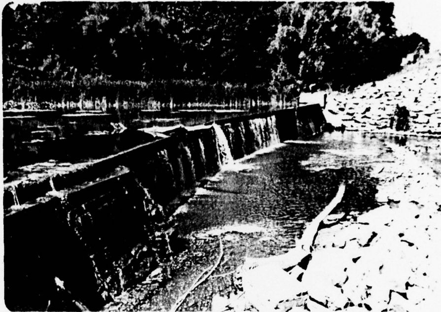
5. Overview of another dam located one mile upstream.
