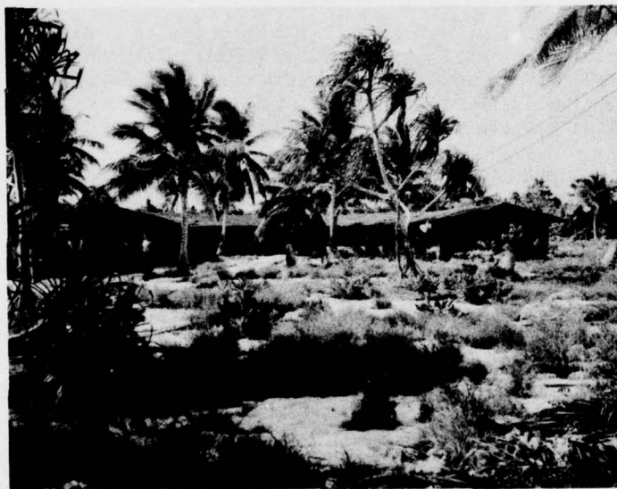
Figure 30. Old Officers' Club on Bikini Island rehabilitated as a SeaBee bunkhouse. ABCR Photo No. 5011-6.
