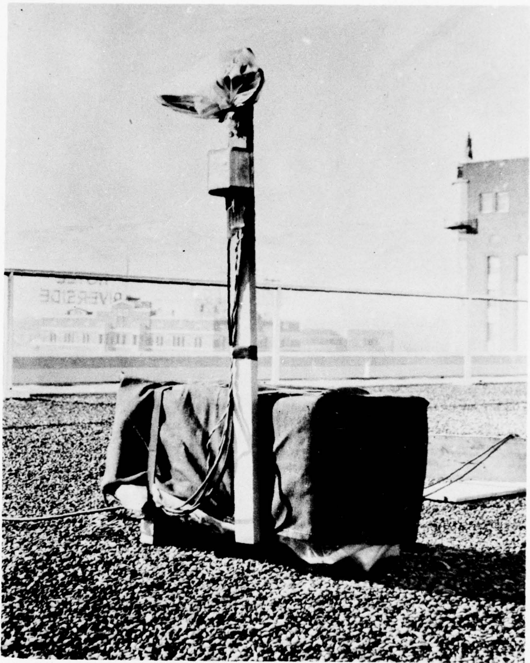
Fig. 1 — Typical radiation-monitoring station installation.
