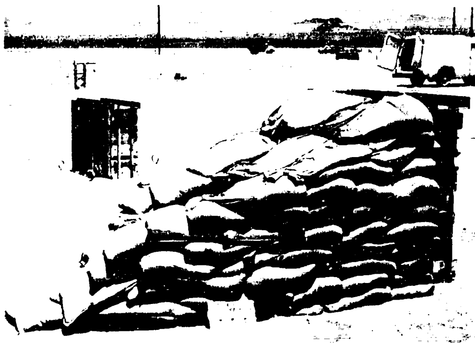
Fig. 2.4 Sandbagging behind forward trap.
