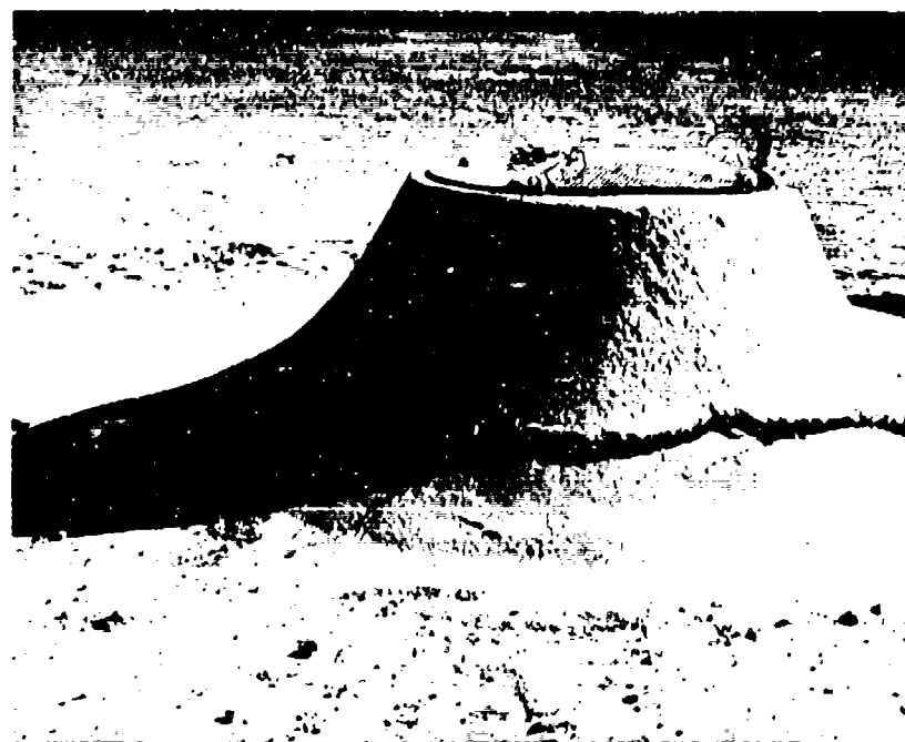
Fig. 3.2b—Damage to aerodynamic mound above shelter 8002.
