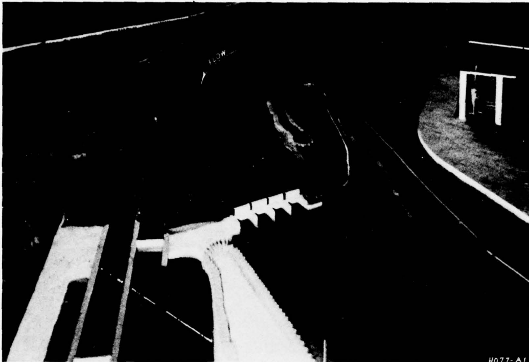
a. Path of downbound 1,200-ft tow approaching lock
