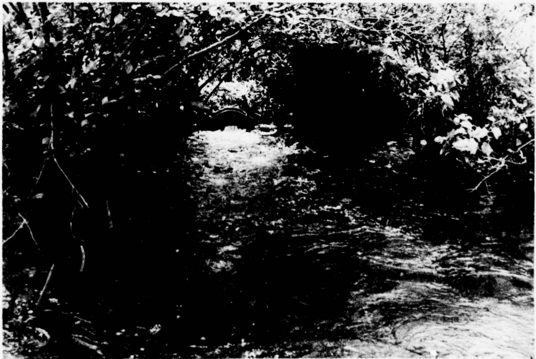
PHOTO 4. Principal Spillway Outlet, Overgrowth, and Stilling Basin
