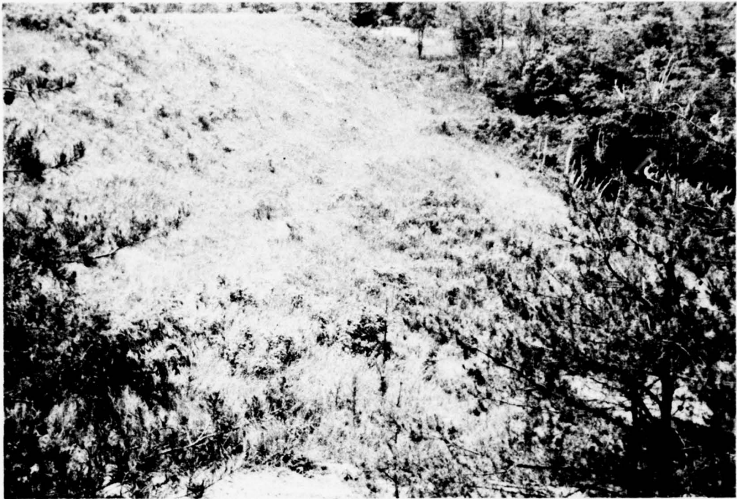
PHOTO 1. View of Downstream Embankment from Right Side of Dam
