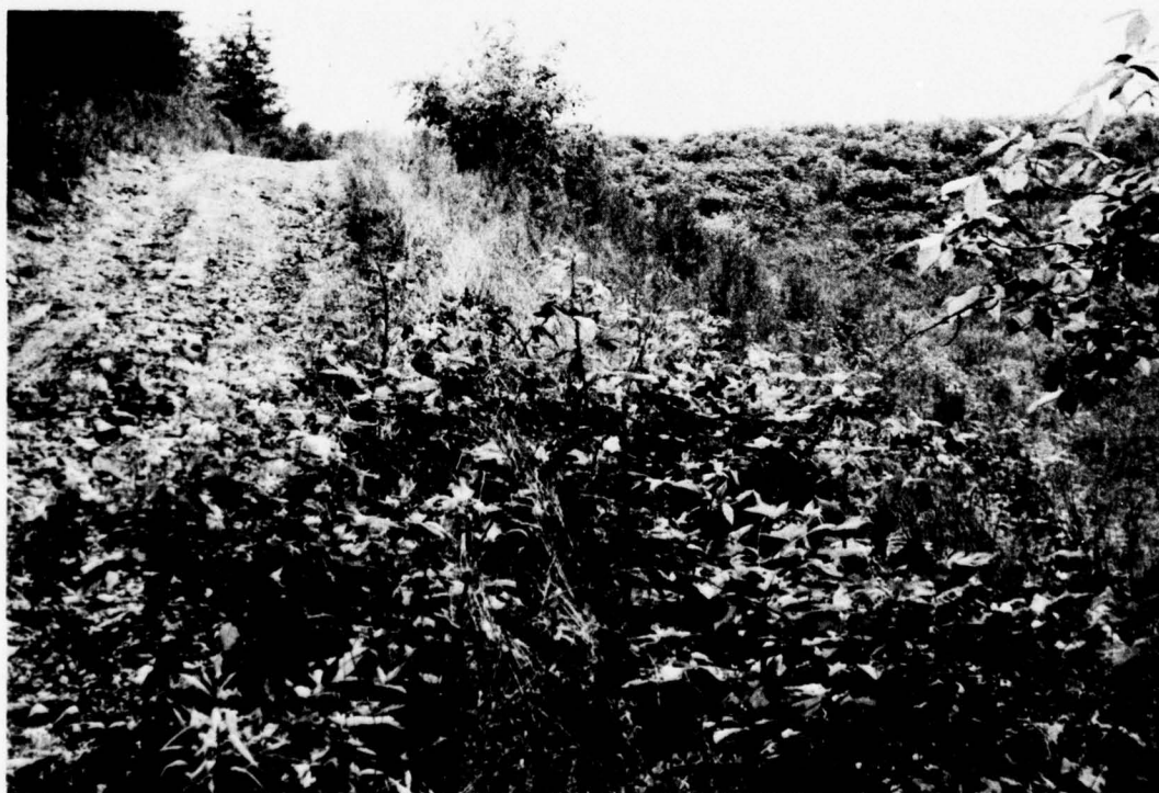
PHOTO 6. Discharge Channel of Right Emergency Spillway Looking Upstream
