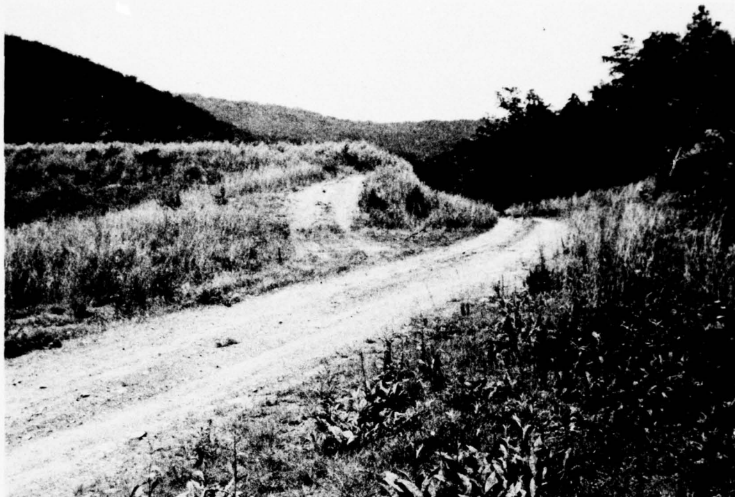
PHOTO 5. Upstream View of Left Emergency Spillway
