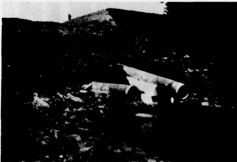
8. Detail of discharge pipes; left pipe draw-down, right pipe principal spillway for multi-purpose pool. Notice small drain pipe on left of pipes.
