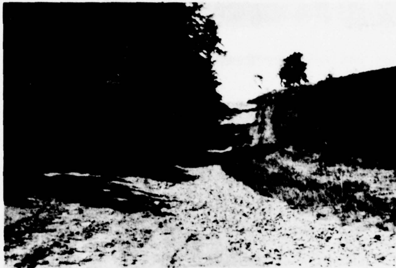
5. Downstream embankment at west abutment. Stone-filled trench at west abutment carries surface drainage and treated effluent from sewage treatment facility.
