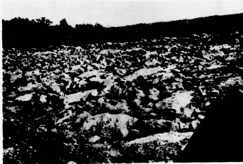
4. Detail of riprap on face of dam.
