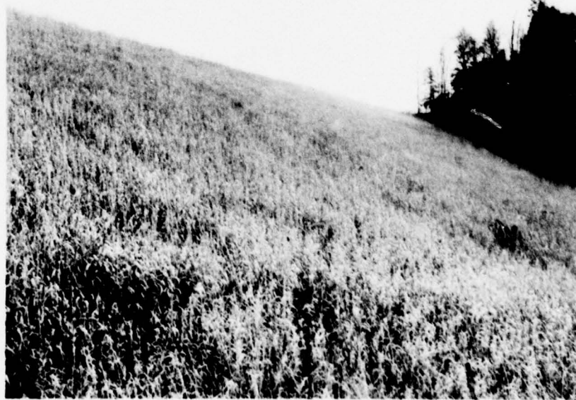
DOWNSTREAM SLOPE OF NORTHERN EMBANKMENT
