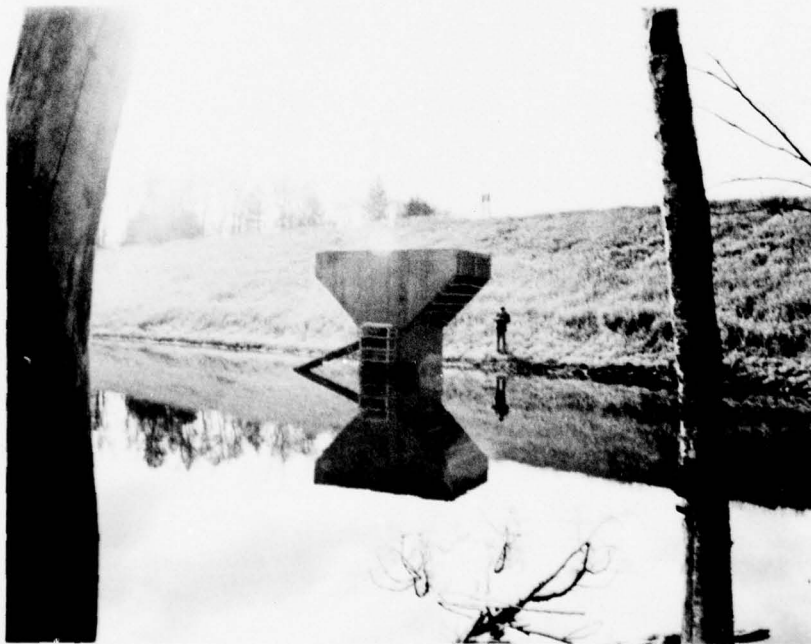
RISER - NOTE LOG LODGED IN TRASH RACK
