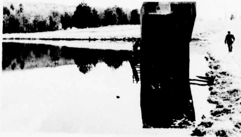
RISER - PRINCIPAL SPILLWAY INLET
