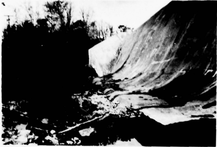
Spillway Looking North
