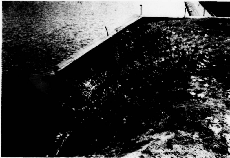
Upstream Face of Embankment Looking South
