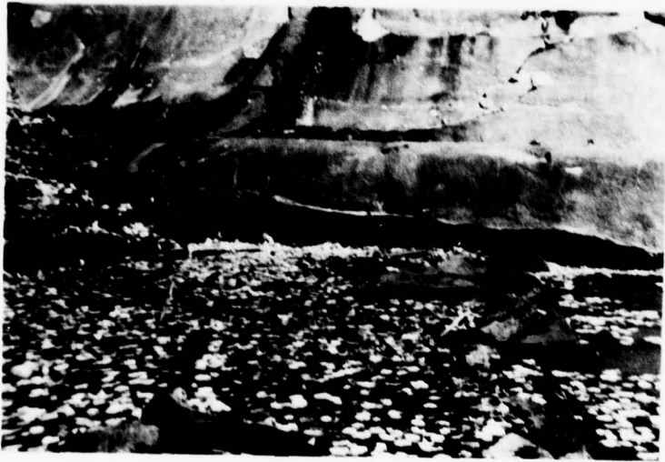
Base of Spillway
