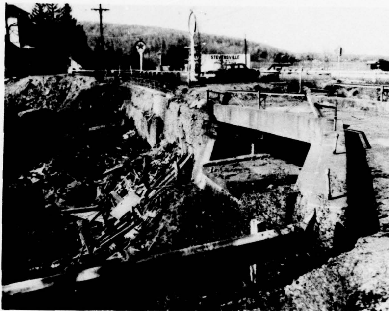
DOWNSTREAM FACE OF DAM (1962) Looking West
