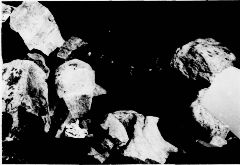
Void under north wall of spillway
