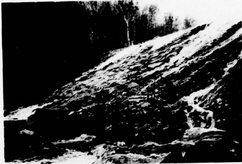
Downstream face of dam Looking North
