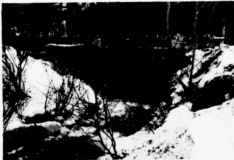
Downstream Channel - Bridge NY Rts 10 & 29A
