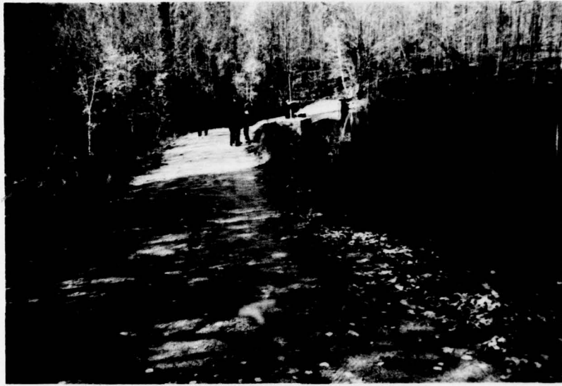
Top of Dam Looking North
