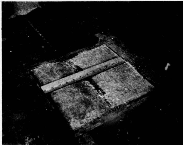
Figure 5. Typical concrete surface condition after the reinforcing steel was lowered. The indentation above the bar is visible.
