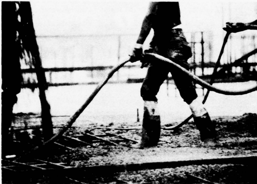
Figure 3. Large vibrator was being used. Its contact with steel would cause the steel to vibrate.
