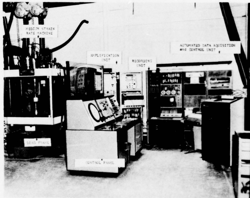
Figure A-1. Automated materials characterization system.
