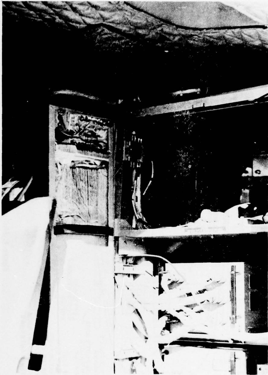
Photo 5. Mission Equipment Cabinets.
