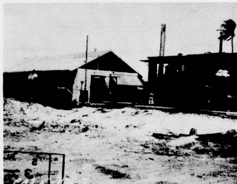
Laundry facilities on Eniwetok Island. This laundry was operated by the Engineer Troops.
