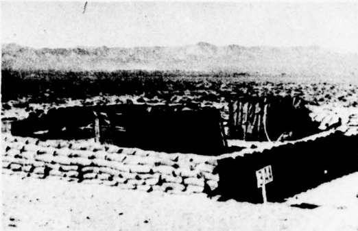
Can vas tank (left rear) of this water purification unit burned at 2500 yds.
