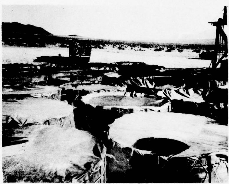
Camp water storage point with a capacity of 120,000 gallons. All water had to be hauled 23 miles.
