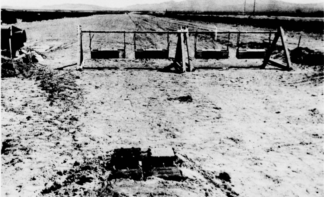
Fig. 4.15 Typical Camera Installation
