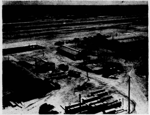
Constructing Plane Wash Rack.
