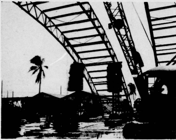
Raising Arc Into Position at B-50 Hangar.
