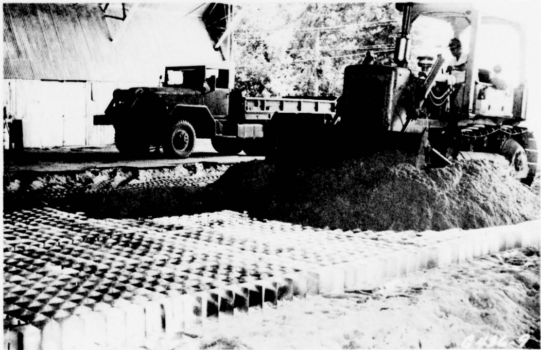
Photo 6. Tractor pushing sand forward into grid cells, test section 1
