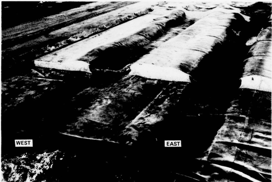
Photo 61. Section view of item 5 after surfacing sand and top membrane were removed at 3500 passes, test section 2
