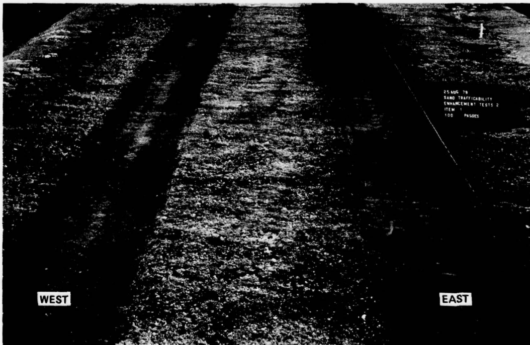
Photo 44. Item 1 after 100 passes, test section 2
