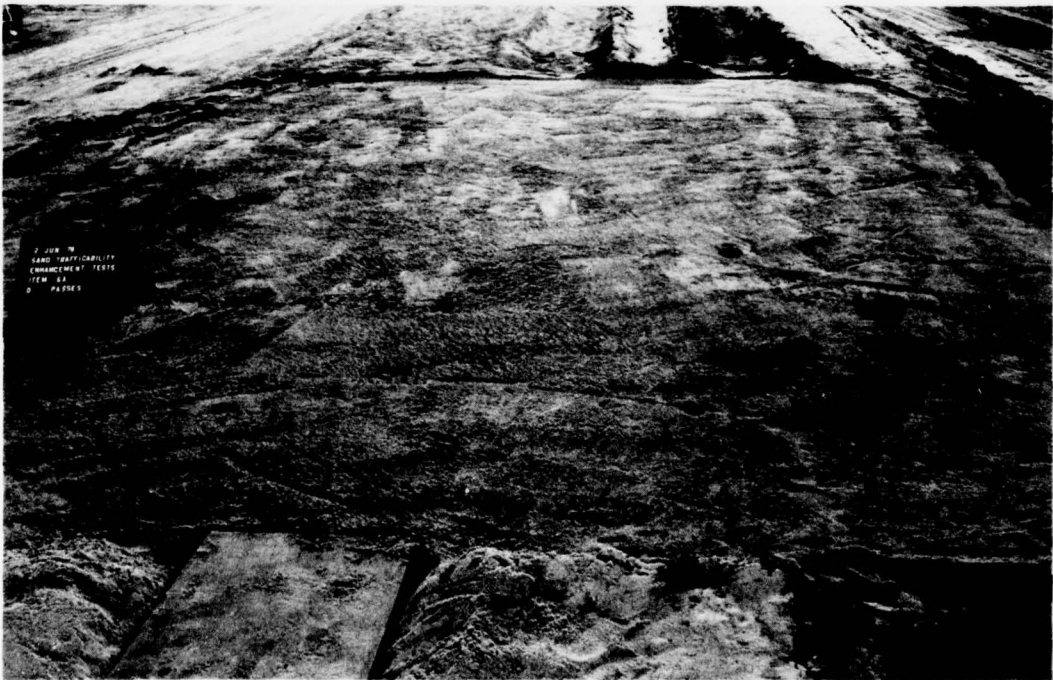
Photo 32. Item 6A prior to traffic, test section 1
