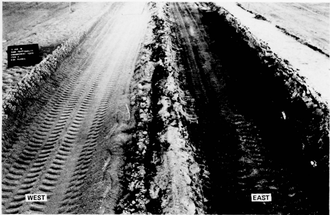
Photo 23. Item 4 after 500 passes, test section 1
