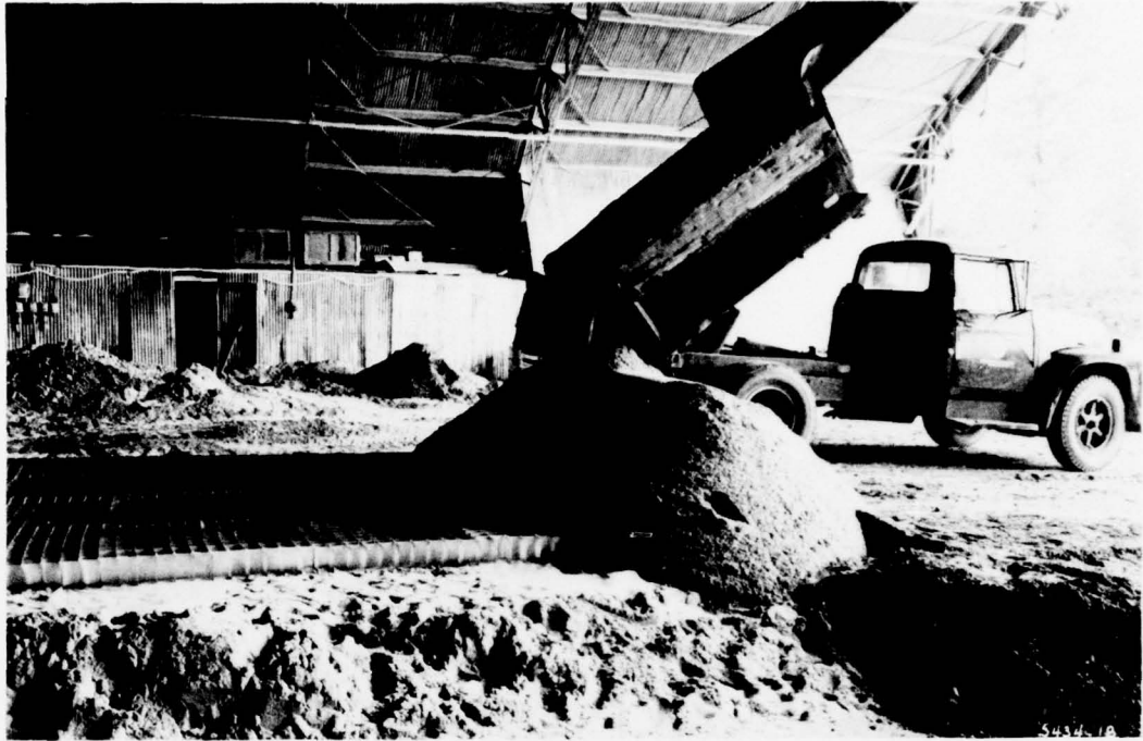
Photo 5. End dumping sand on grids, test section 1
