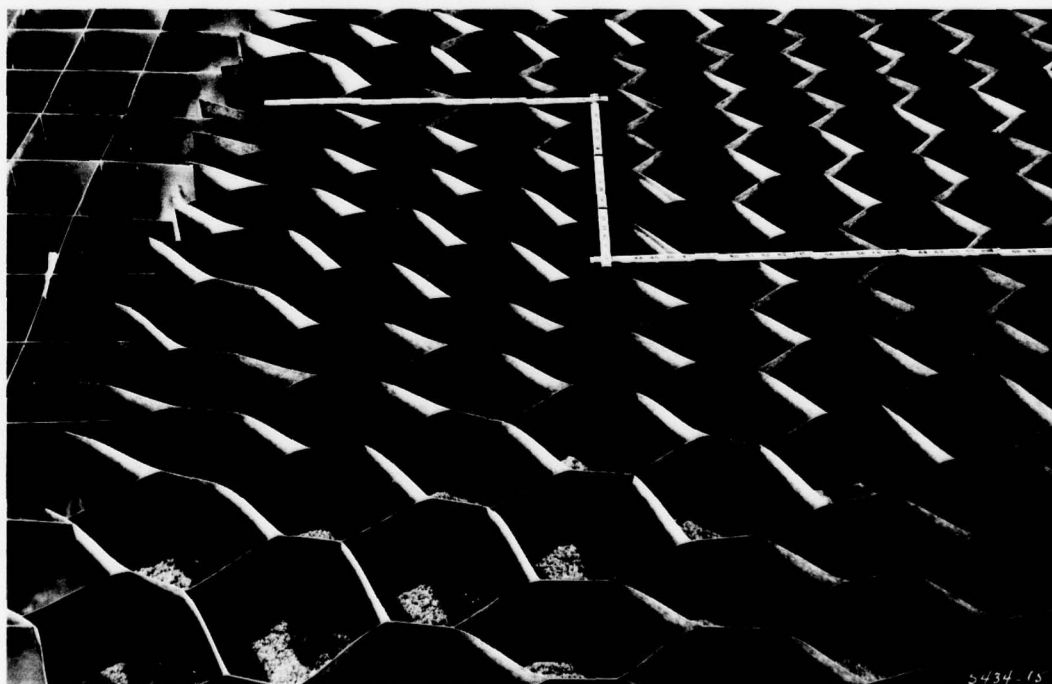
Photo 10. Closeup view of 8-in. Hexcel paper grids, item 5, test section 1
