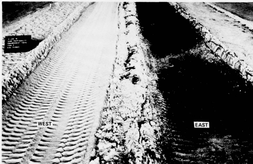
Photo 20. Item 2 after 500 passes, test section 1
