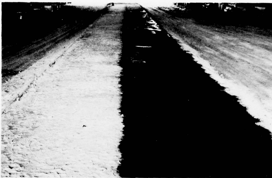
Photo 15. Overall view showing asphalt penetration after 24 hr, test section 1
