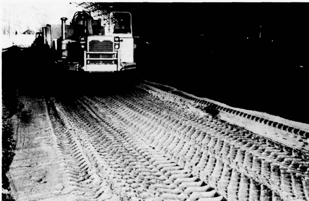
Photo 9. Compacting sand-grid layer using towed-type rubber-tired roller, test section 1
