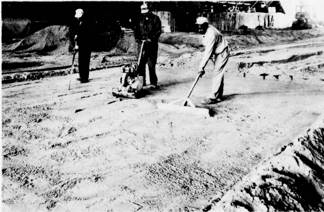
Photo 12. Leveling and compacting base layer of sand, item 7, test section 1
