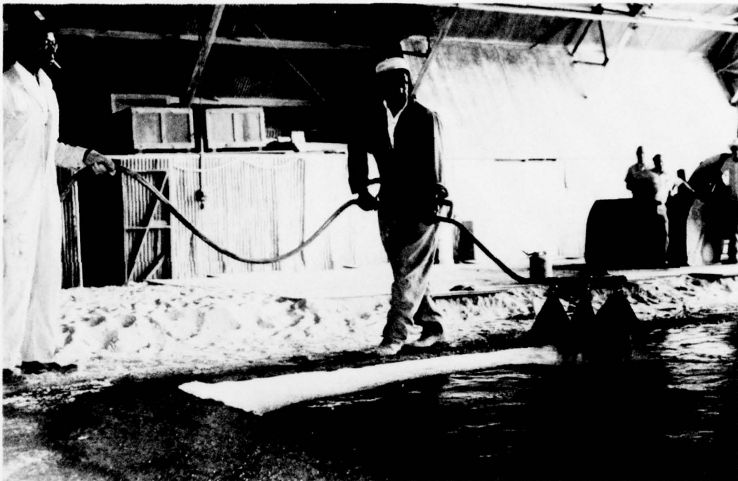
Photo 39. Spraying SS-1 asphalt on fabric, item 1, test section 2
