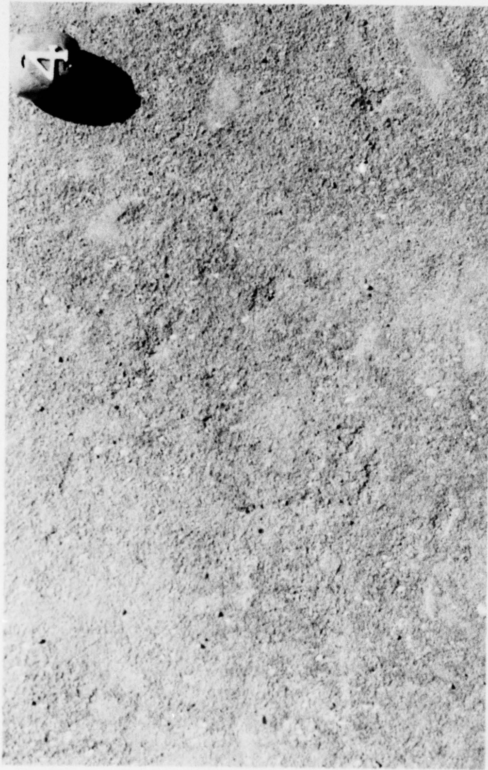
Photo 15. Surface texture of item 4 (second concrete placement lane) after compaction
