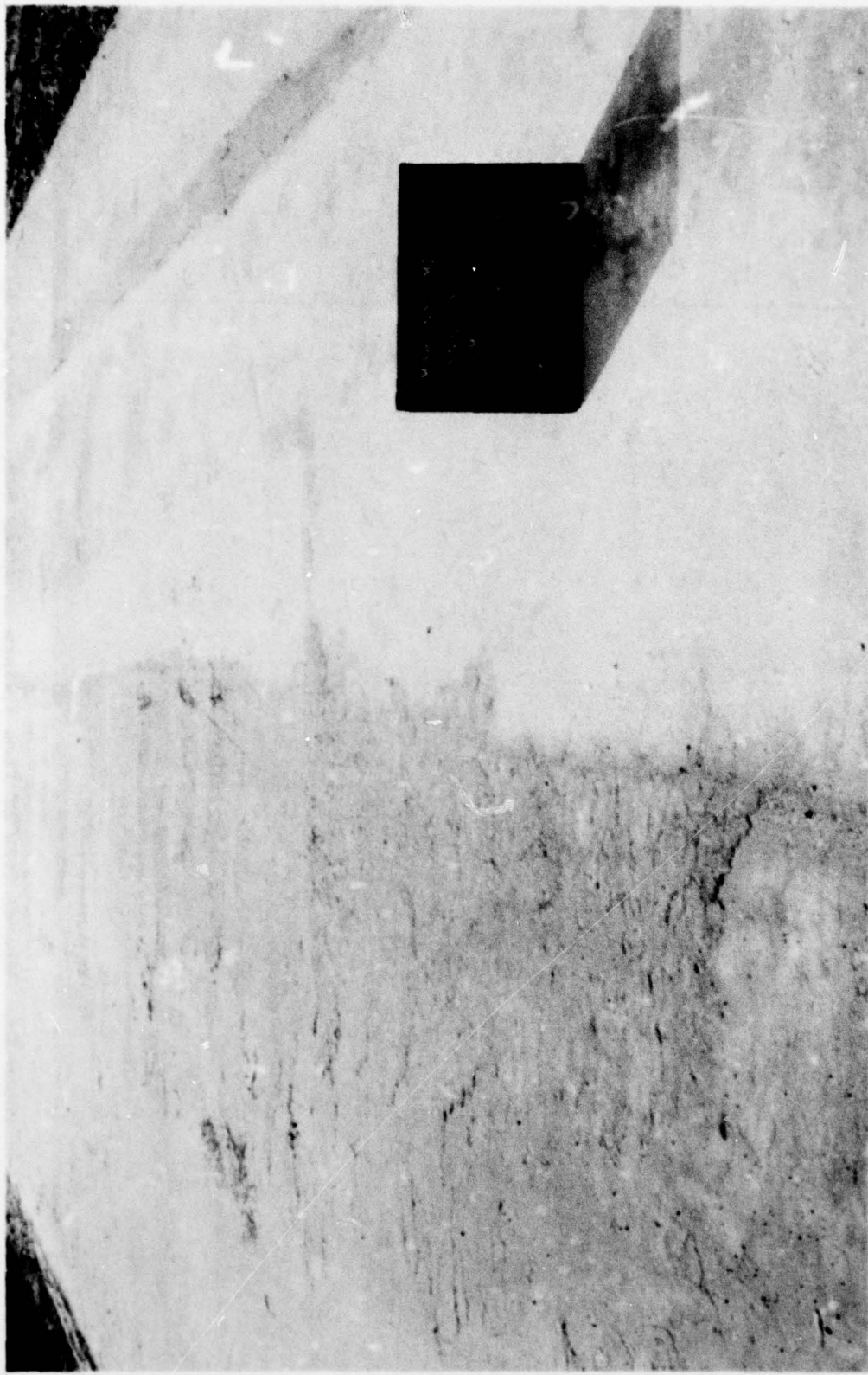
Photo 71. General view of item 3 (rigid pavement) prior to traffic
