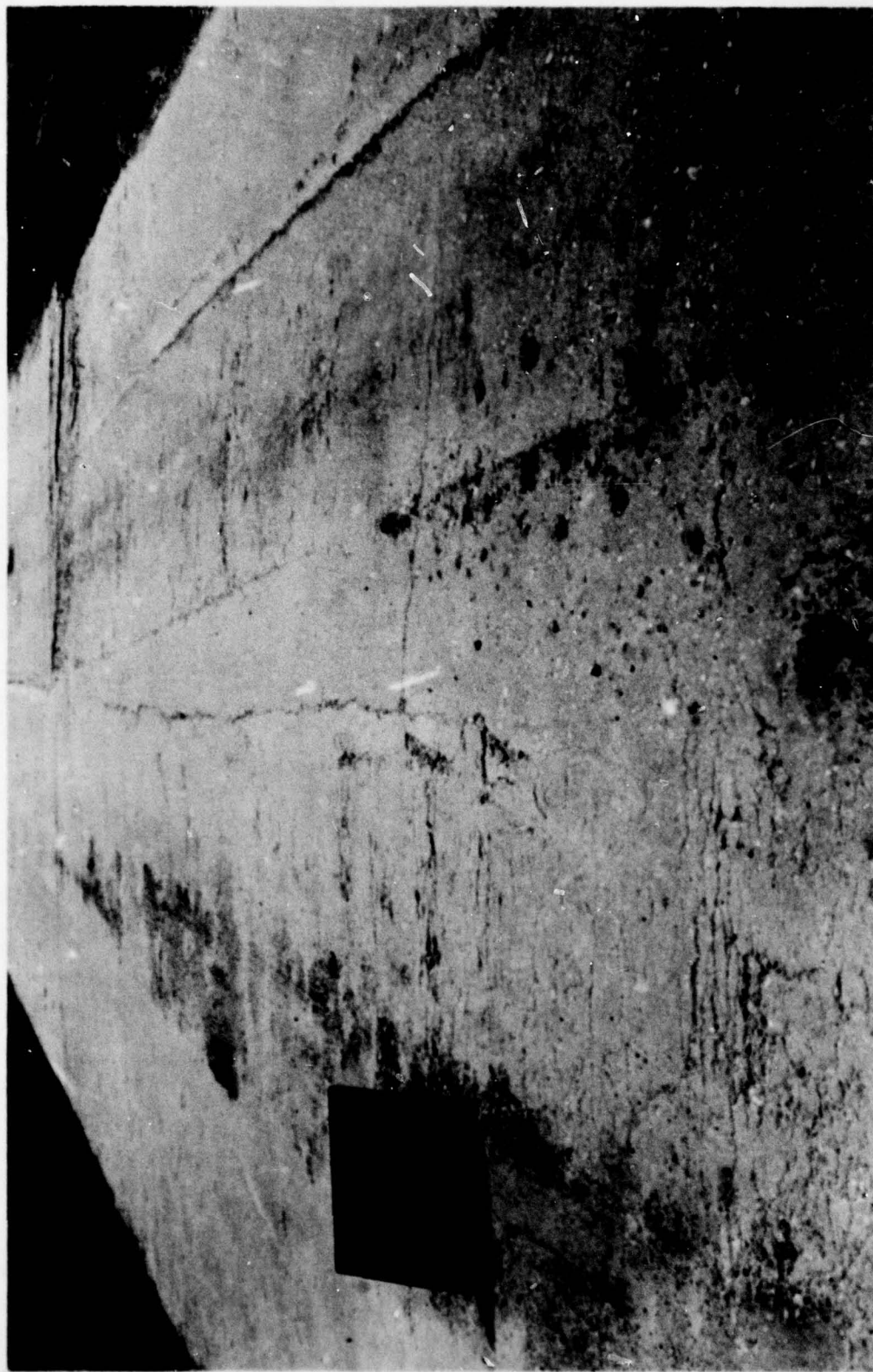
Photo 72. General view of item 3, lane 1, after 125,000 operations
