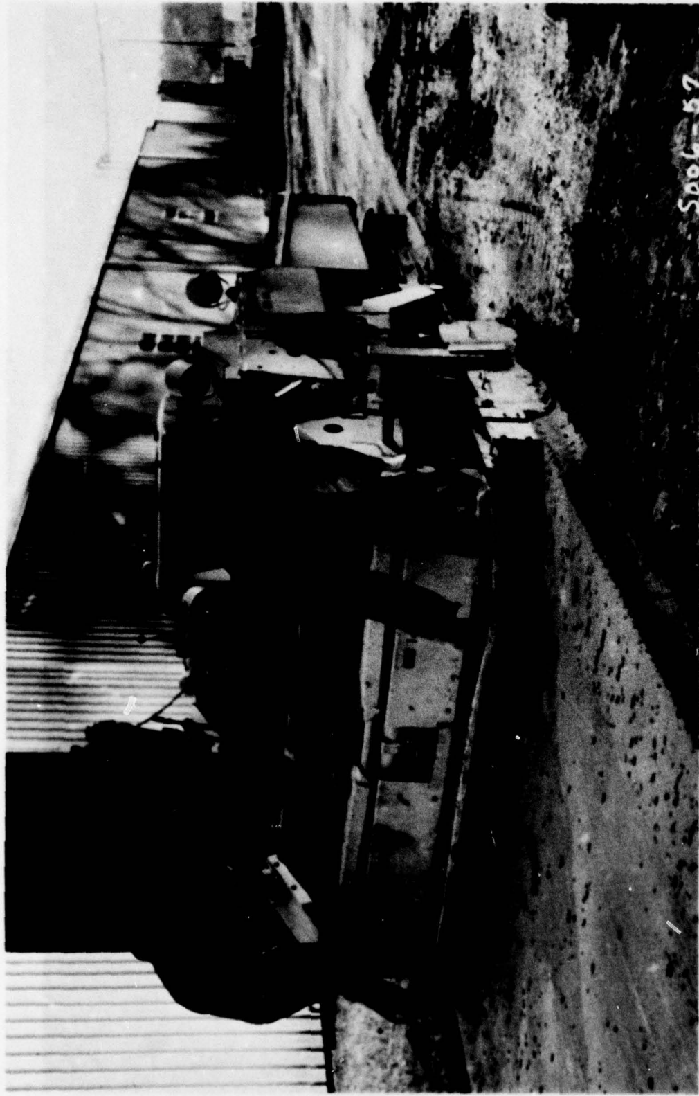
Photo 9. Placement of zero-slump mix with an asphalt finisher
