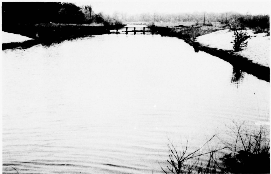
Figure 4. Straight approach channel viewed from pumping station (trashrack in background)
