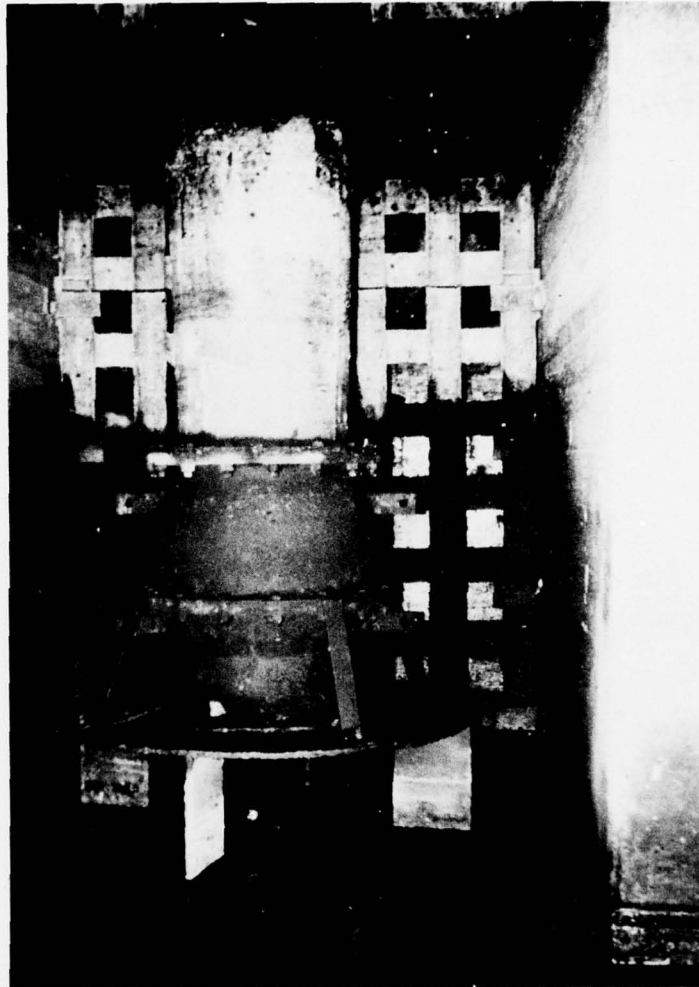
Figure 23. Vanes to straighten flow into the pump intake and a vertical grid on the back wall to attenuate vortex development
