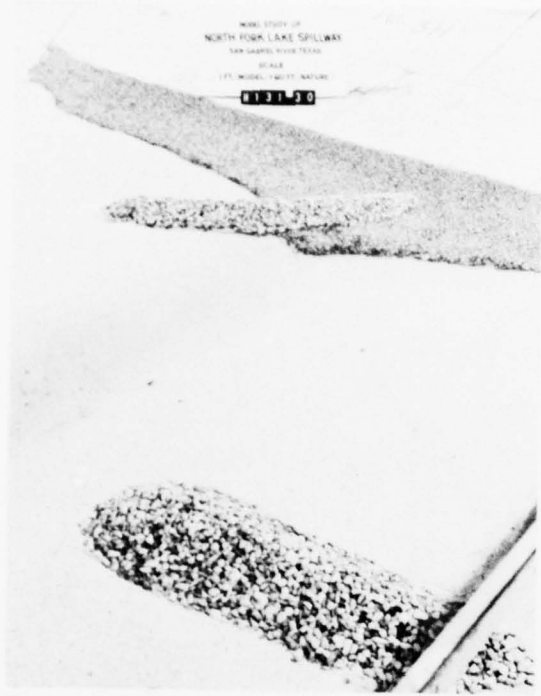
a. Closeup view
