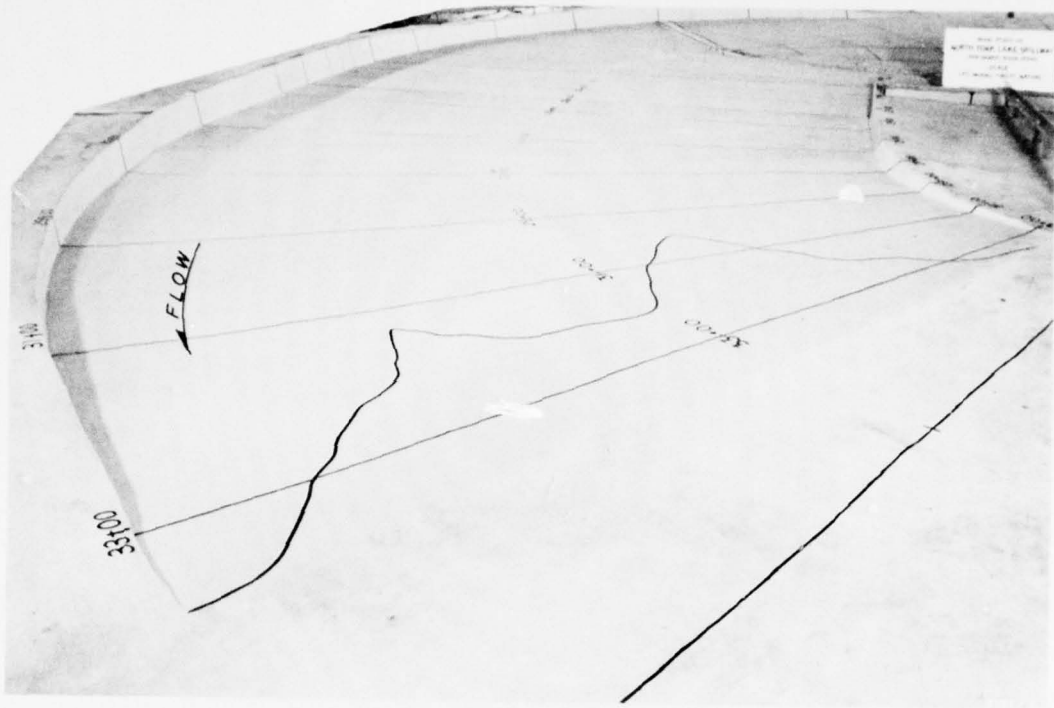
c. Downstream spillway and discharge channel
