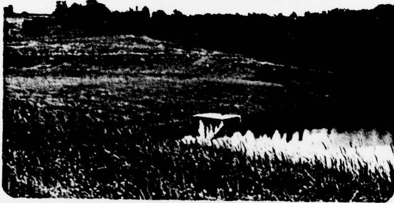
C. Main Spillway and Auxiliary Spillway Approach Channel
