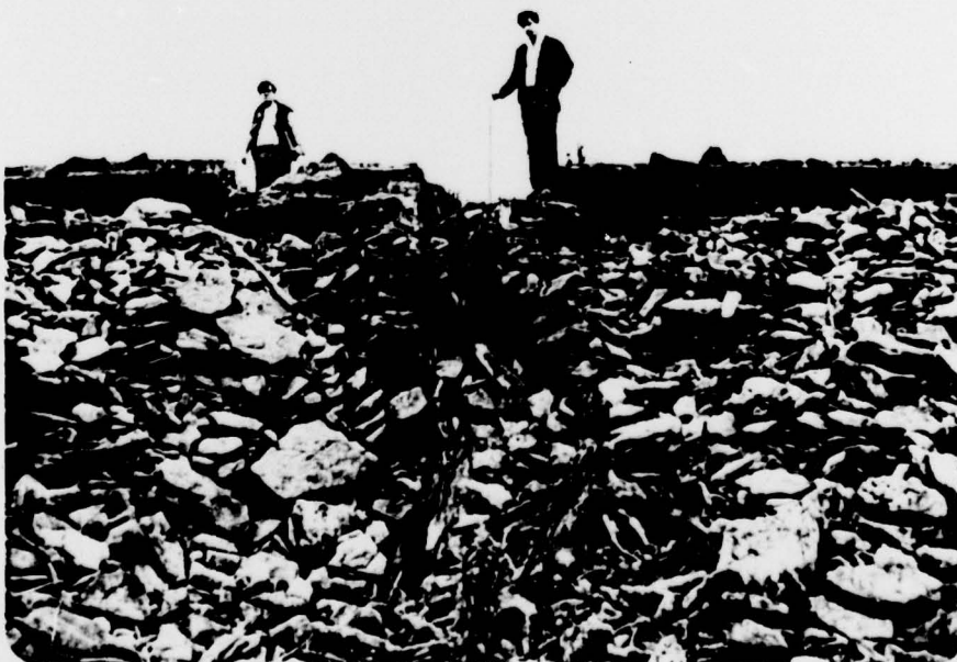
D. Washout Near Ice Chute
