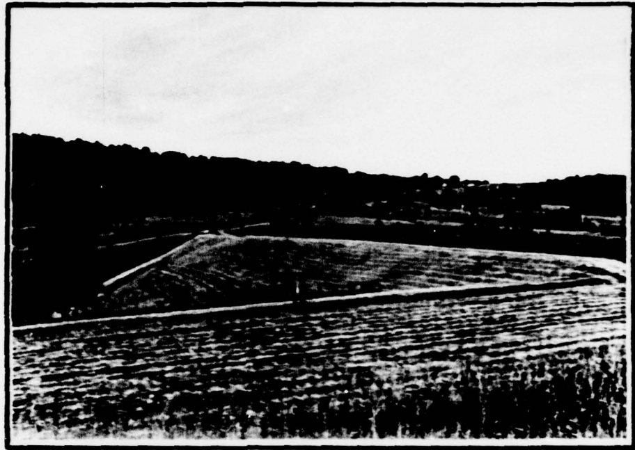
Overview of downstream slope of dam.
