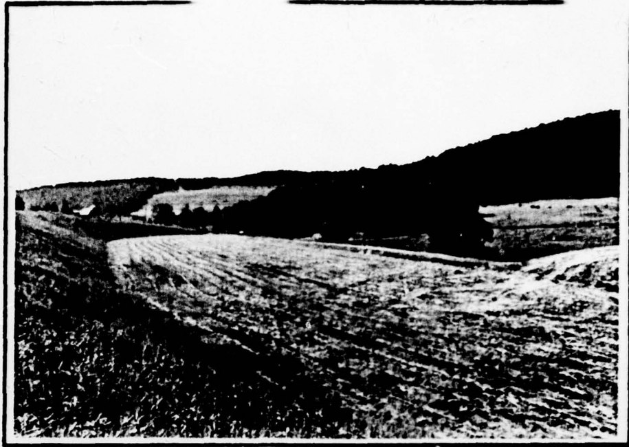
Emergency spillway discharge channel. Note low spot on right berm.
