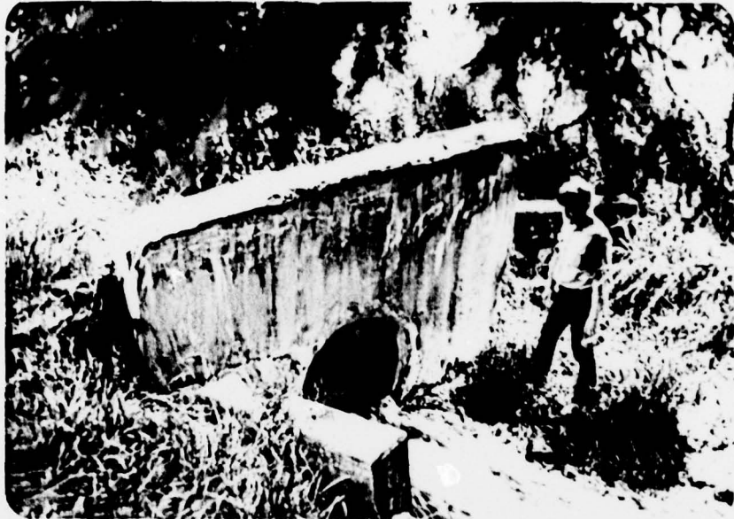
E. Headwall at Conduit Outlet.
