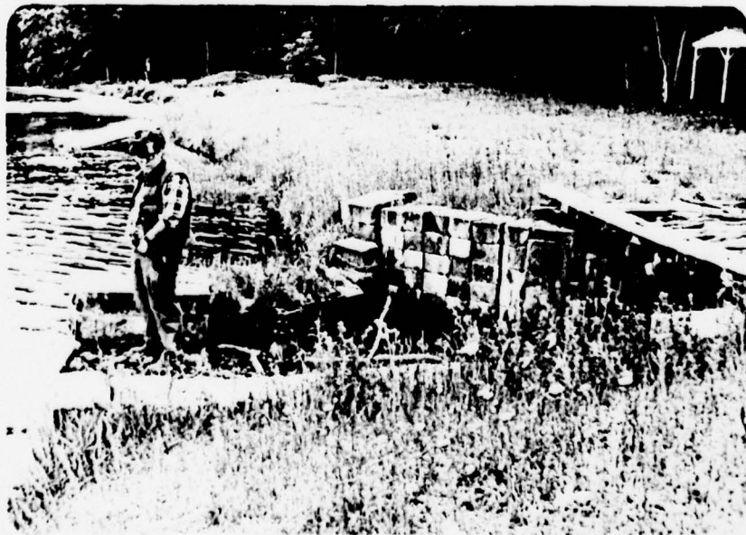
K. Spillway Structure at Pine View Dam.
