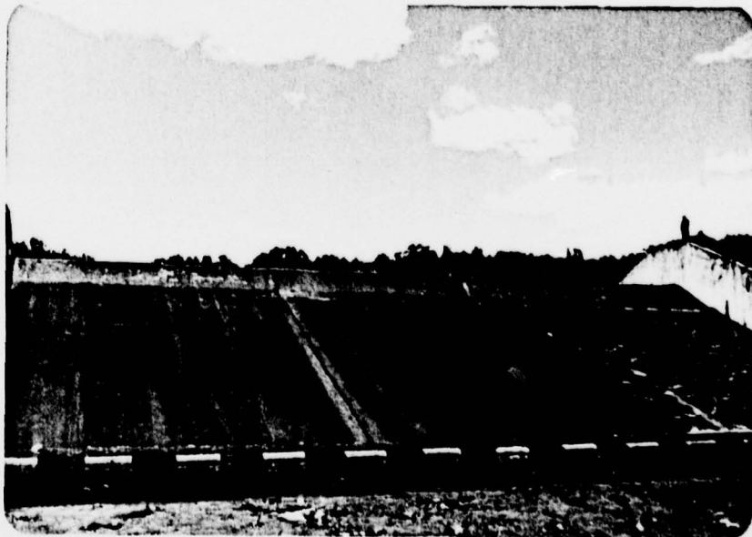
F. Spillway Chute and Stilling Basin.
