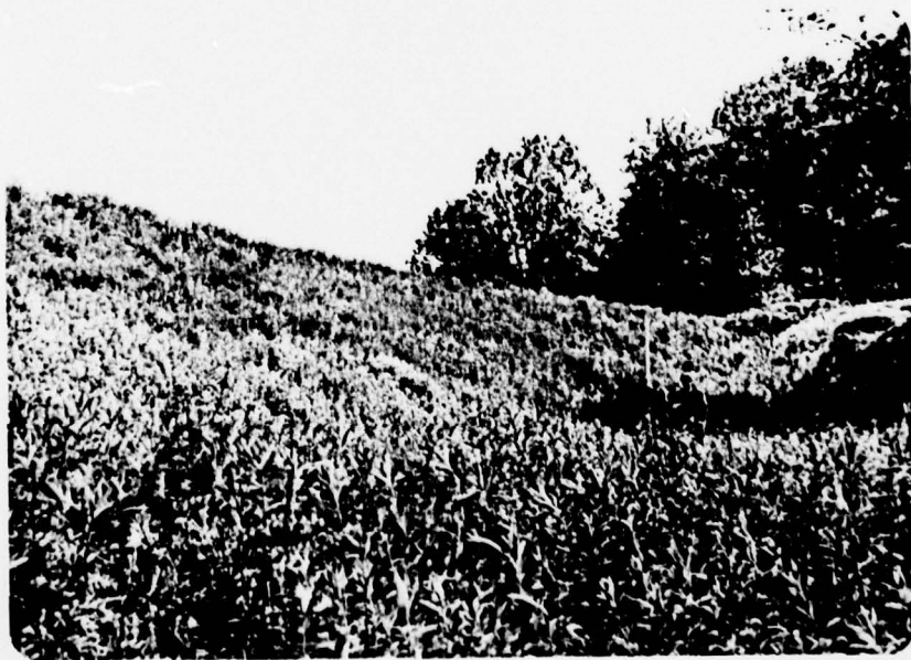
B. Downstream Slope and Left Abutment.
