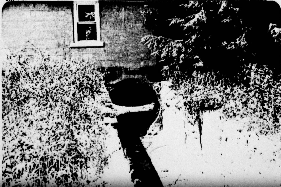
Bypass Conduit Gate at No. 2 Dam
