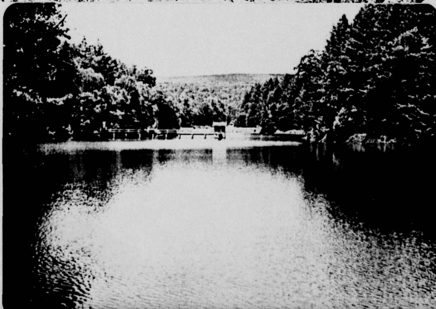
Dam No.4 Reservoir with Submerged No.1 Dam and No.2 Spillway
