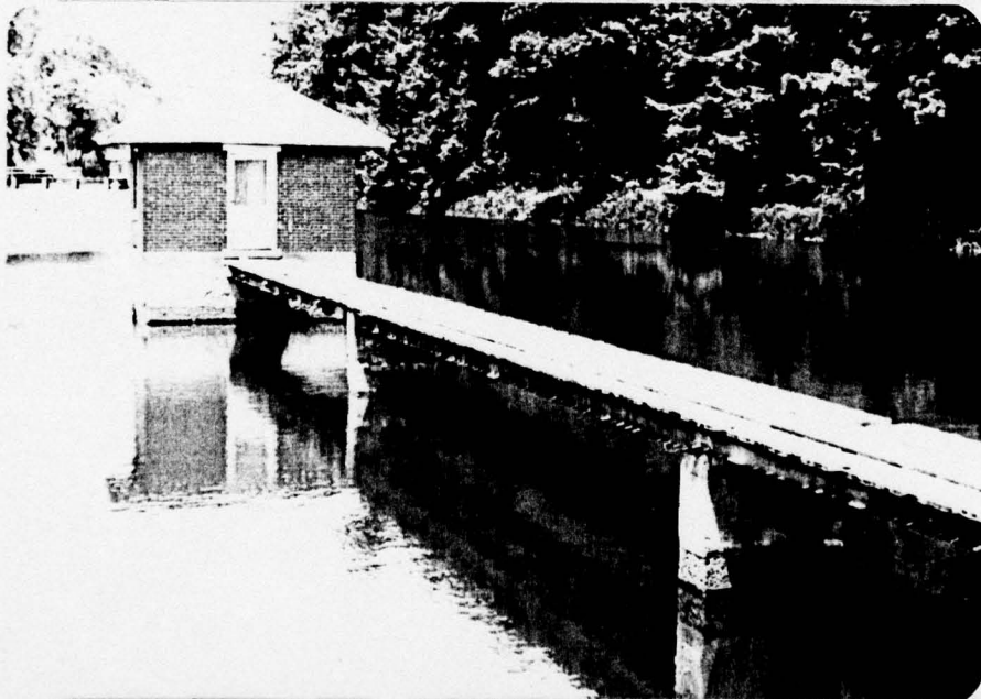
Footbridge to Intake Structure
