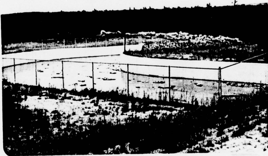
Curved Spillway Discharge Channel
