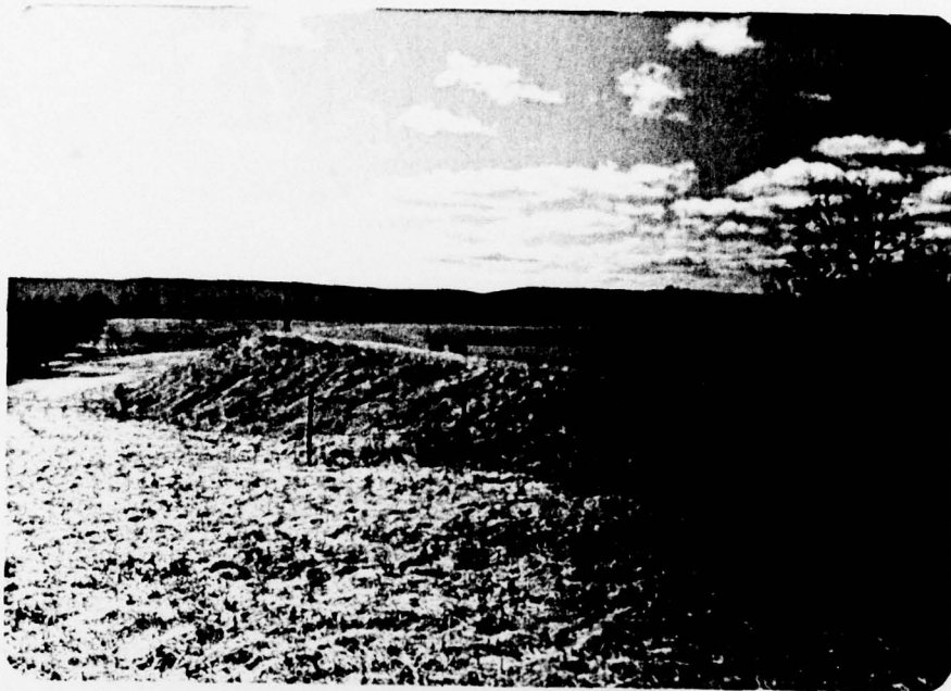
A. Downstream Slope
