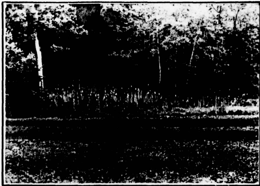
Wet area at downstream toe.
