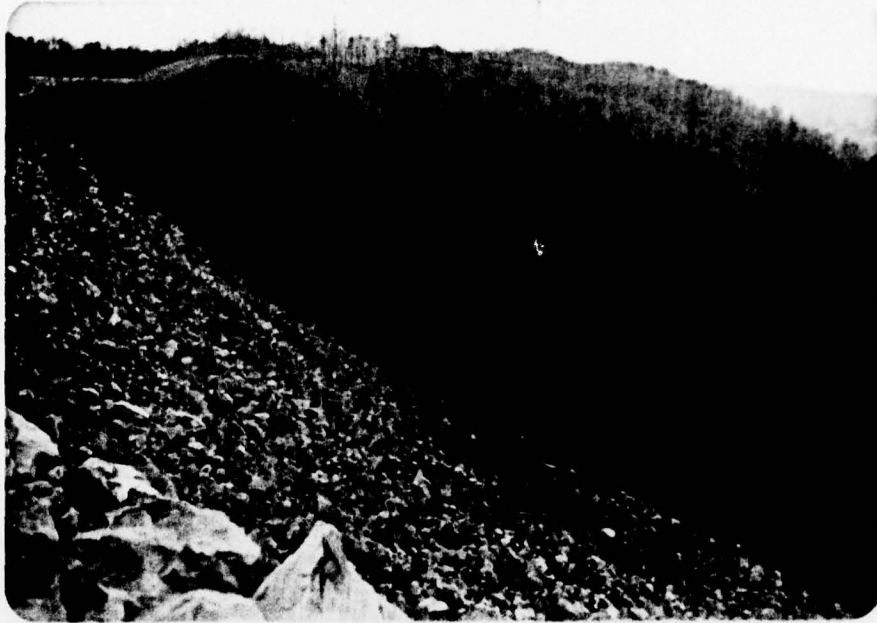
Photograph No. 5 Left abutment. View from crest.
