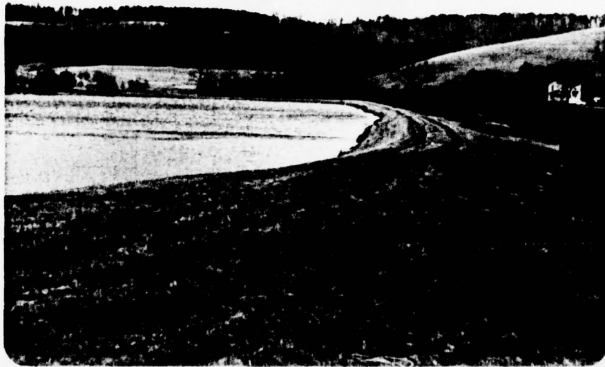
Photograph No. 1 Crest (looking east).
