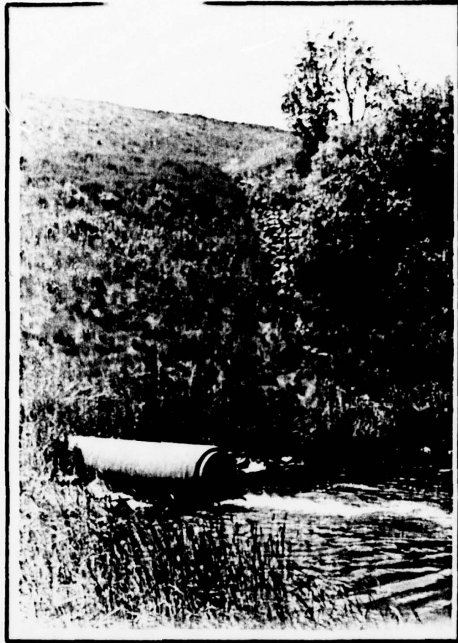
Outlet works and principal spillway discharge.
