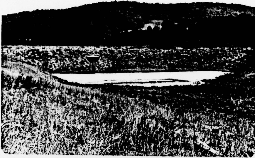
A. Upstream Slope of Embankment.
