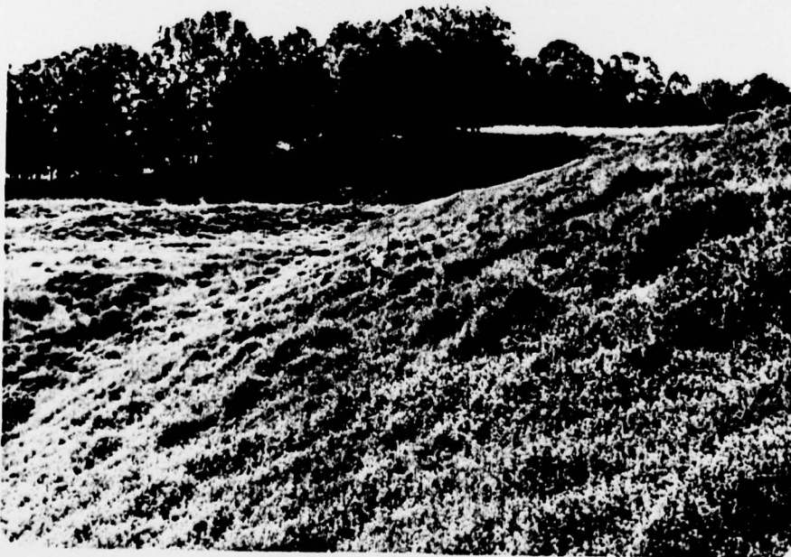
B. Downstream Slope of Embankment.
