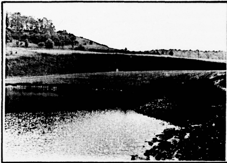
Spillway approach channel.
