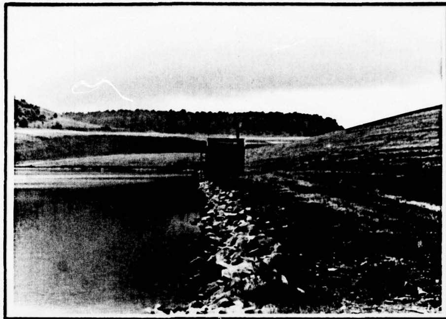
Principal spillway, orifice invert and drain line structure.
