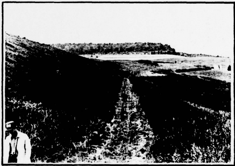
Downstream slope of dam.
