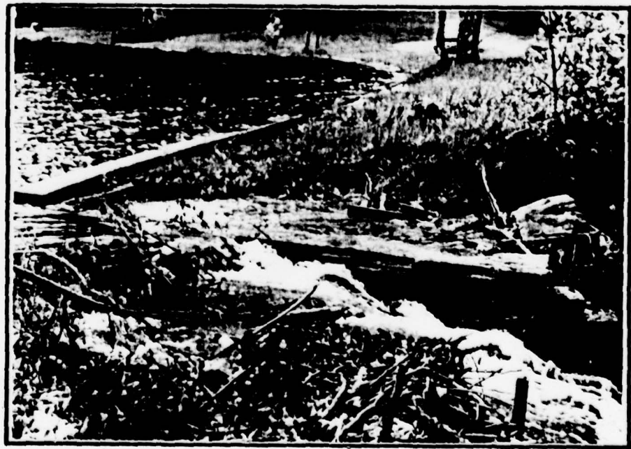
Debris blocking spillway and water flowing around spillway.
